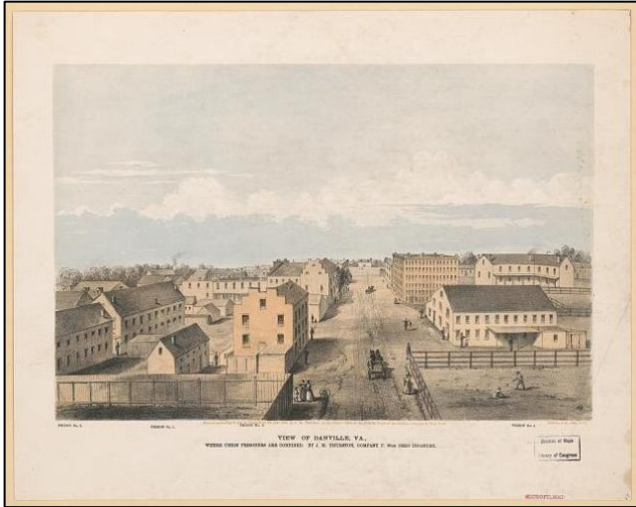
Danville's Prisons (Courtesy of the Library of Virginia)
